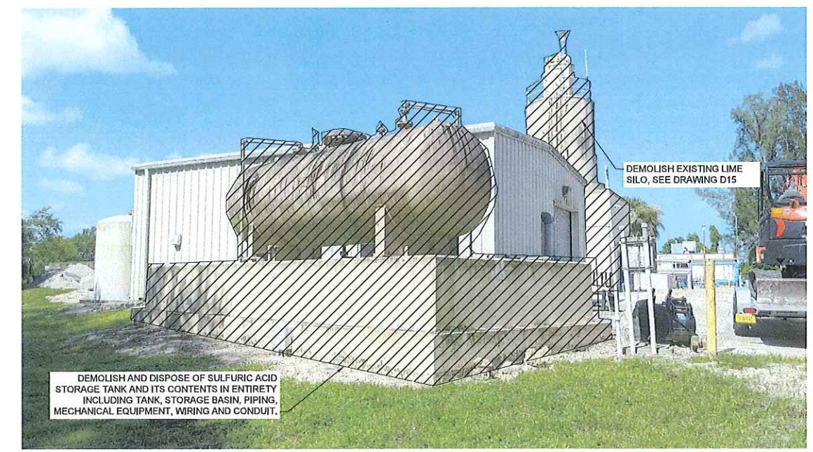
T PHOTO FILE: SULFURIC ACID STORAGE TANK-1
