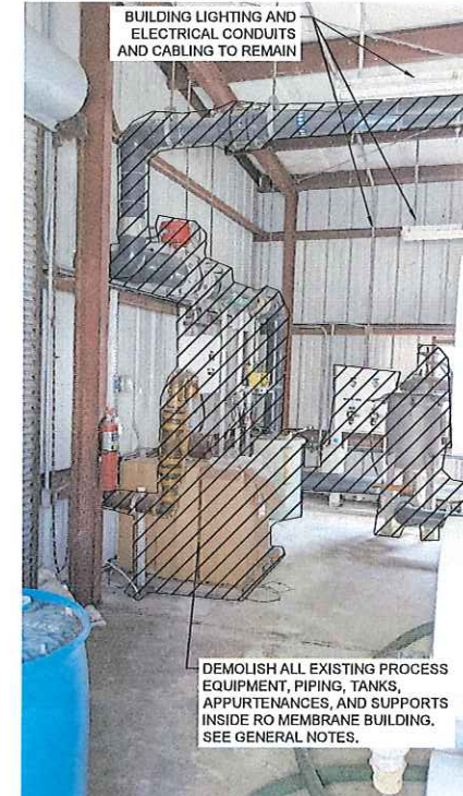
DEMOLISH ALL EXISTING PROCESS EQUIPMENT, PIPING, TANKS, APPURTENANCES, AND SUPPORTS INSIDE RO MEMBRANE BUILDING. SEE GENERAL NOTES.
